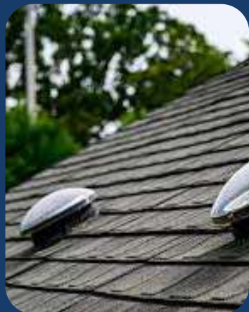
Natural light tunnels
