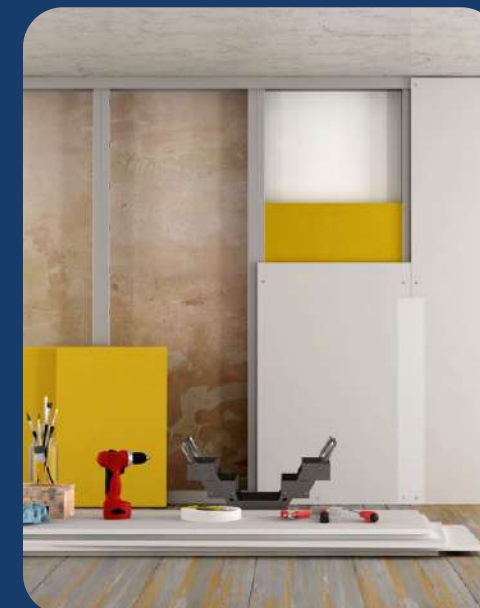
Additional wall reinforcement
