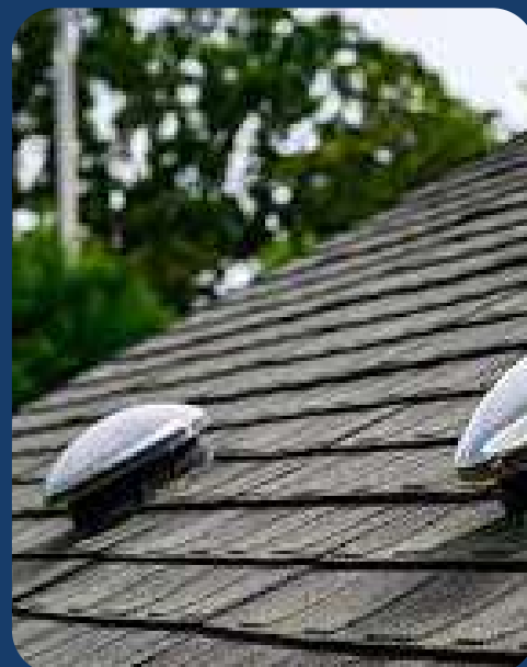
Natural light tunnels
