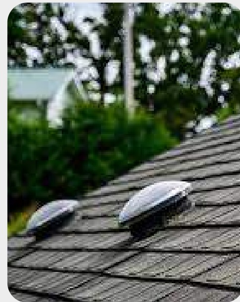
Natural light tunnels
