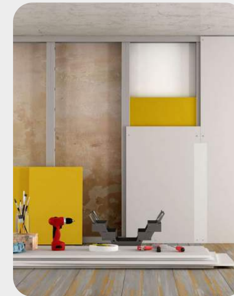
Additional wall reinforcement
