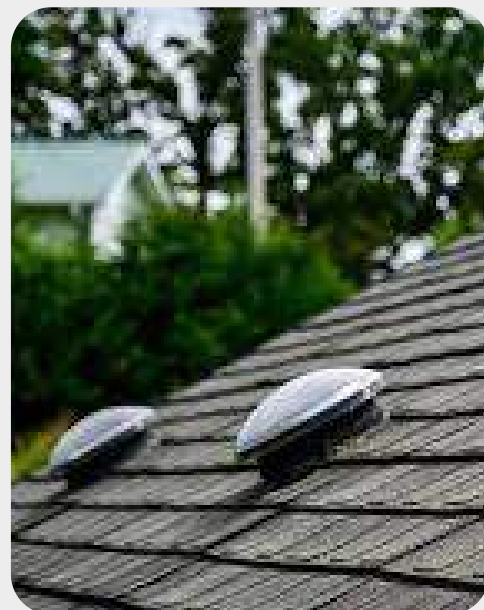
Natural light tunnels
