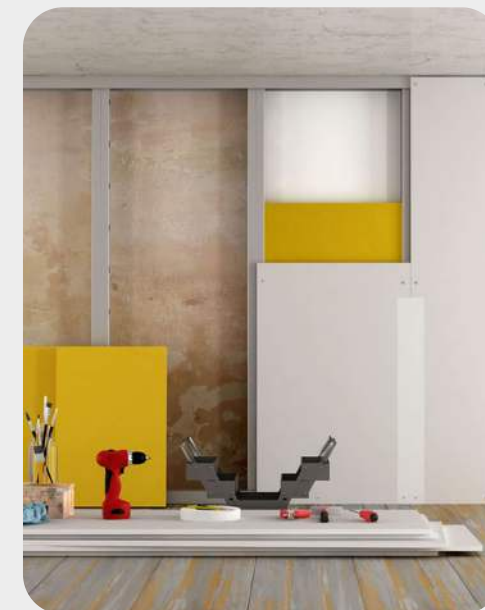
Additional wall reinforcement
